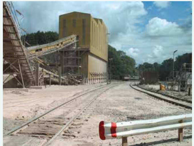
Rail terminal for handling crushed carboniferous limestone at Whatley Quarry
